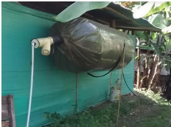
Figure 8. Chorizo-type biodigester implemented in Villa Letty / Biodigestor tipo chorizo implementado en Villa Letty
